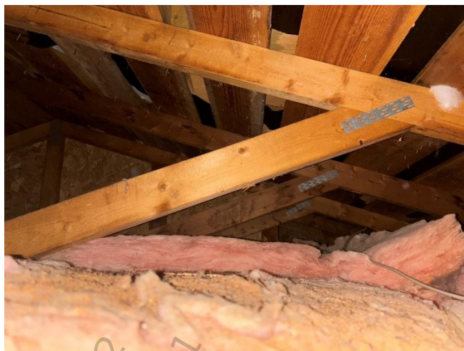
Photo 1: Typical roof structure.
