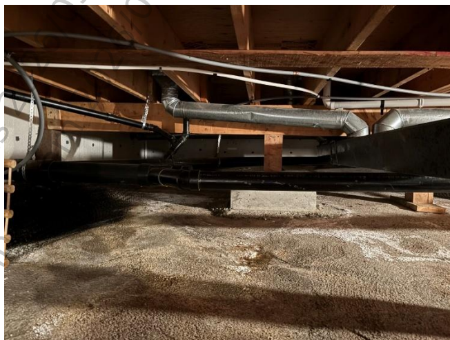
Photo 2: Typical crawlspace with limited clearance.
