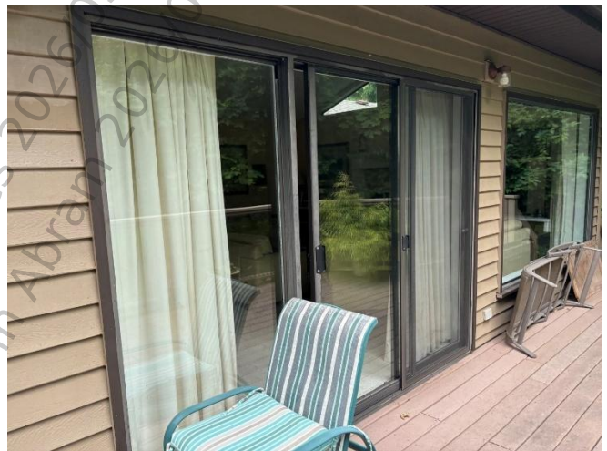
Photo 10: Typical sliding door at main deck.
