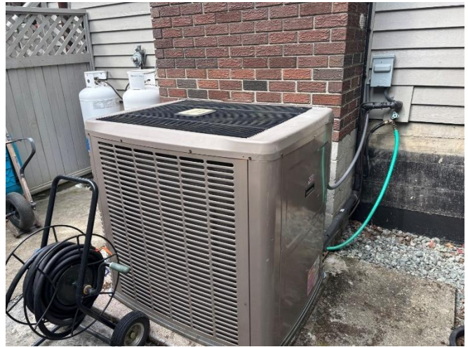
Photo 29: Typical heat pump.
