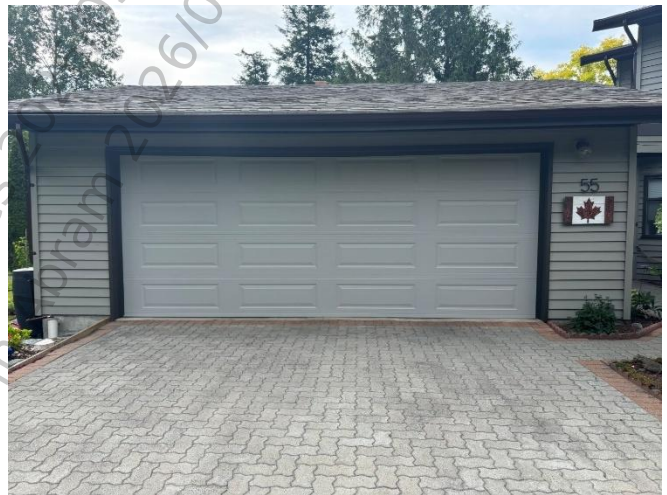
Photo 12: Typical garage door.
