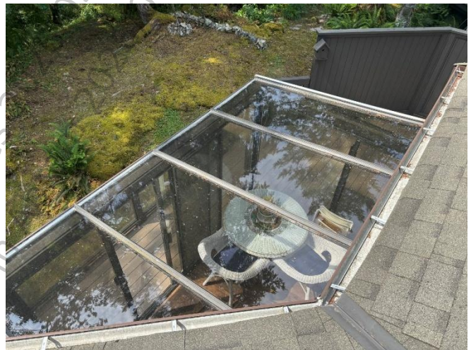
Photo 15: Typical solarium as observed from the roof.
