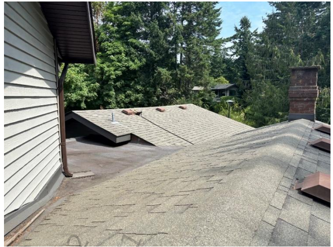
Photo 16: Typical sloped and flat roofing.
