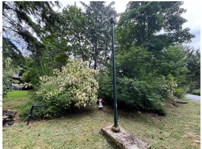
Photo 41: Typical pole-mounted fixture.
