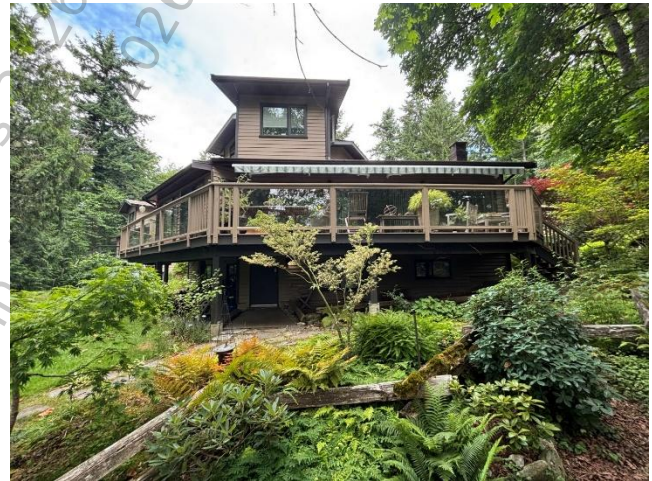
Photo 2: Typical main deck.
