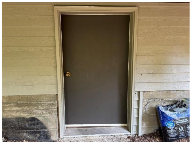
Photo 13: Typical crawl space door.
