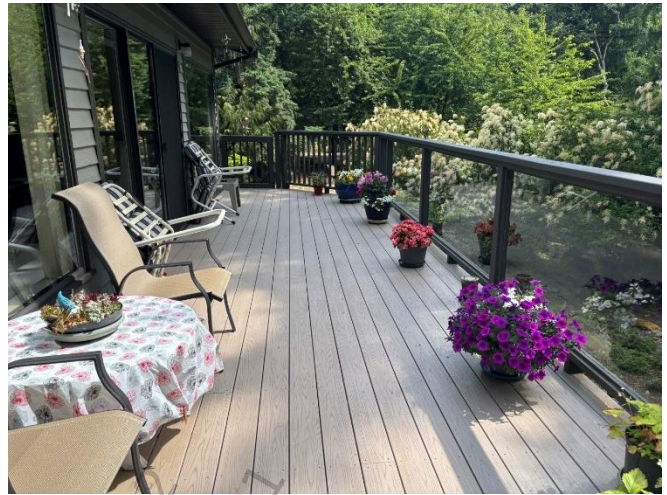
Photo 4: Typical main deck.
