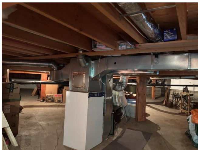
Photo 3: Typical crawlspace with additional clearance.
