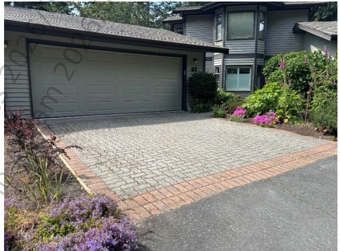
Photo 25: Typical brick-paved driveway.
