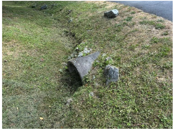
Photo 34: Typical ditch and culvert.
