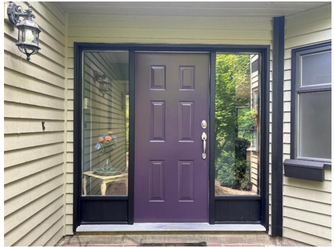
Photo 11: Typical townhouse unit entrance door.
