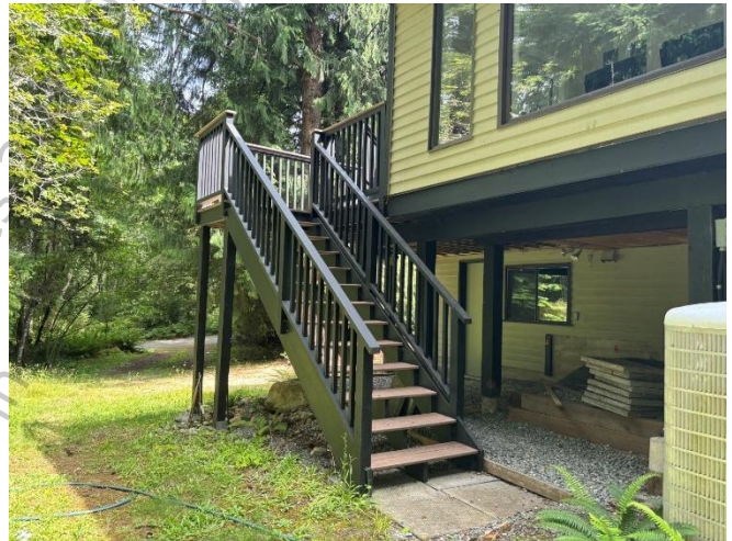
Photo 5: Typical staircase providing access onto main deck and supporting wood posts.
