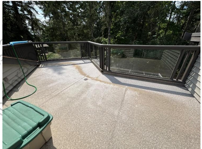
Photo 17: Typical upper deck.
