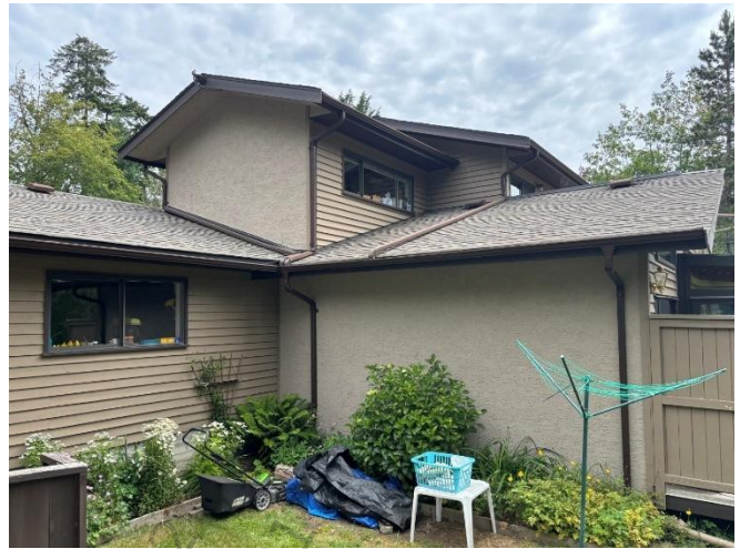
Photo 6: Typical wood siding and stucco cladding.
