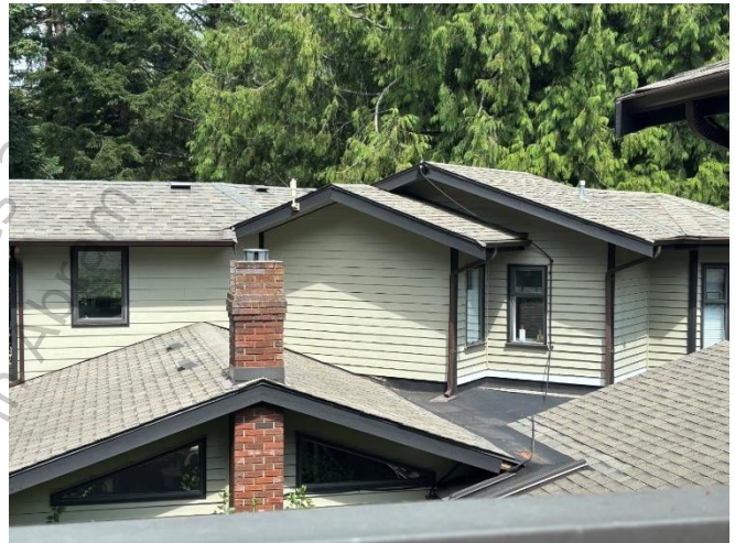
Photo 7: New fibre cement lap siding and typical brick chimney.
