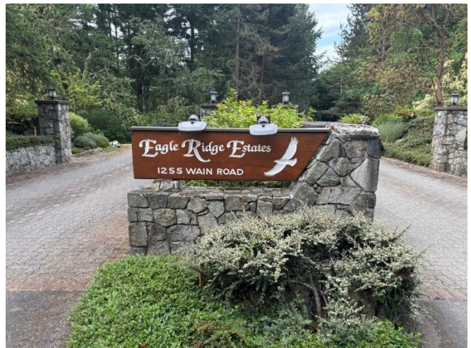
Photo 42: Complex entrance light fixtures.
